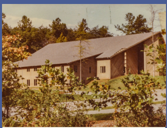
Trinity building under construction, 1982
